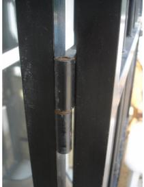
To secure the pins and prevent them being knocked out is relatively simple and was suggest by Rod who is one of the Home watch members. His solution is effectively tamper proof, using "groove pin" known locally as metric roll pins see picture. People need to ask for a 'pasador' (grove pin/roll pin) 4mm and suitable for standard rejas. They can be bought at the car accessory outlet, a little further down from the BP garage on the opposite side.
